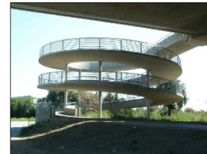
Indicative Spiral ramp example Reinforced concrete construction
